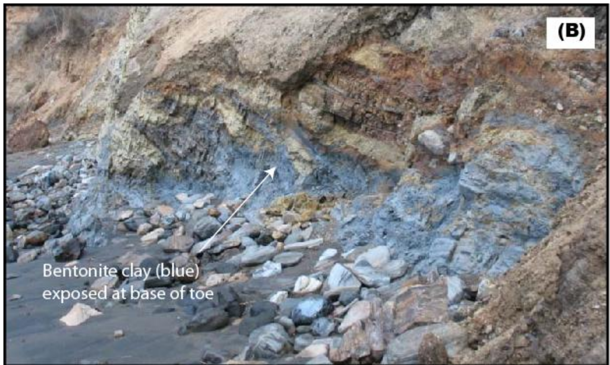
Figure 3.13. Terrestrial analog: Portuguese Bend landslide. (A) Schematic cross section of the Portuguese Bend landslide in Palos Verdes, CA, showing features of the slide (after Kerr and Drew, 1969). Note the clay-rich (altered tuff) layers along the slip surface, which experienced a significant loss in shear strength upon absorption of water and lubricated the base of the earthflow during emplacement. This example provides a mechanistic analog for VM landslide outer zone emplacement, whereby seismic shaking induces thixotropic flow and basal lubrication by smectite clay to form earthflow long runout. (B) Bentonite clay (blue) exposed at the base of the Portuguese Bend landslide toe, revealing its contribution to lubricated basal slip (after Douglas, 2011).
