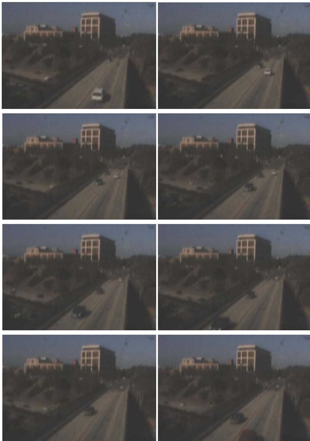
Figure 6.16. Traffic flow crossing over the bridge
