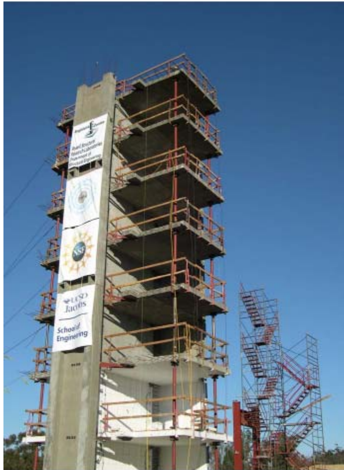
Figure 5.9. Picture of the seven-story shear wall building slice
