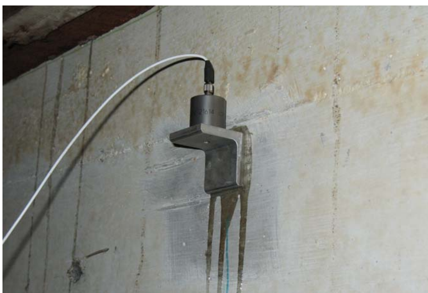
Figure 6.6. Picture of a piezoelectric accelerometer installed on the stem wall
