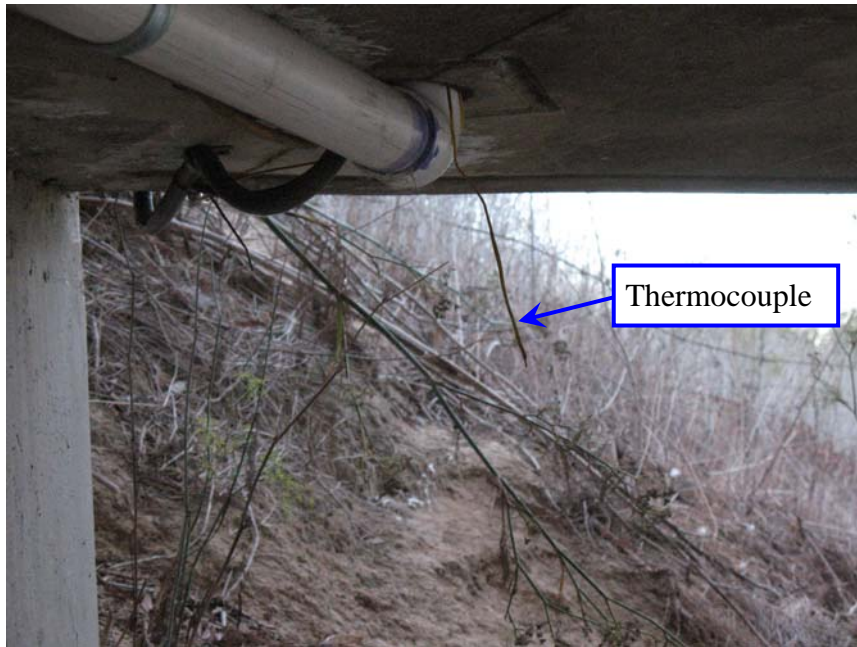
Figure 6.12. Thermocouple used to measure the air temperature underneath the bridge
