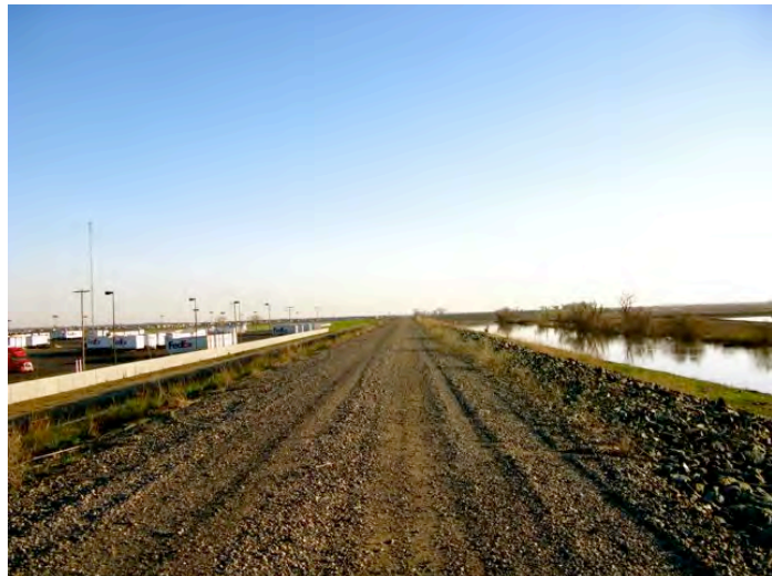
Figure 3. Levee at Lisbon Slough.
