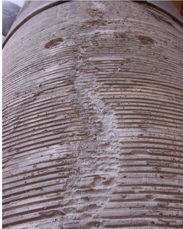
Fig. 5.25 Concrete core at north side of the splice (see Figures 2 and 4)
