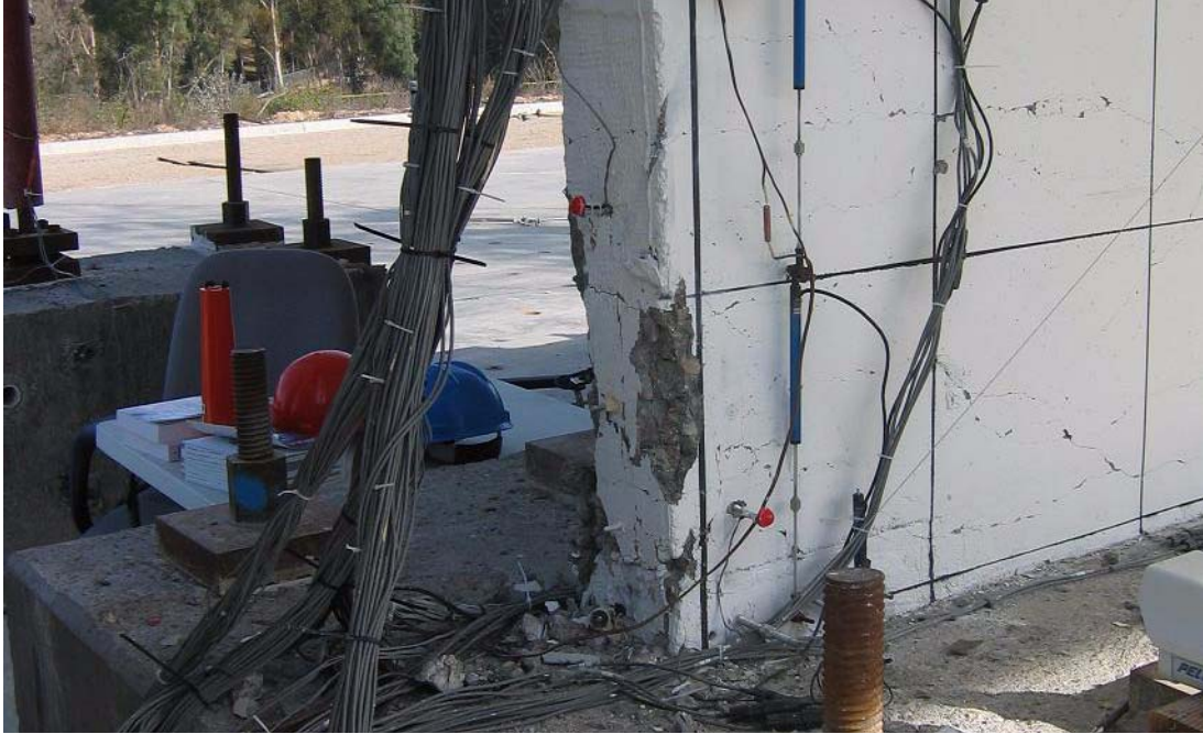
Fig. 6.14 Observed damage at the bottom of the first story of the web wall on the west side at damage state S4
