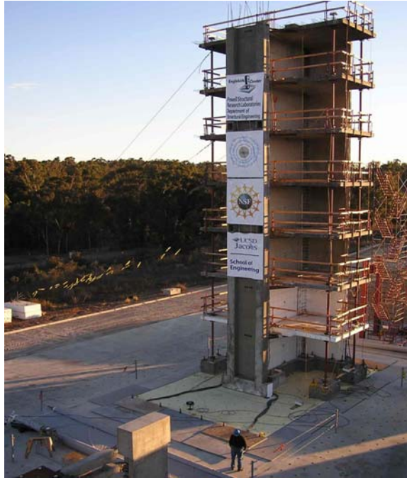
Figure 4.1: Seven-story full-scale R/C building slice, 19.2m high.
