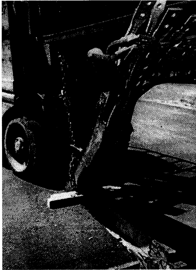
Figure 4.2 Removal of cables to repair thermal expansion buckling
