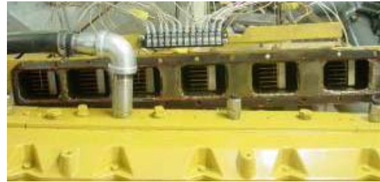
Figure 4 - ICTC Manifold Prior to Installation Showing All Six Port Heaters
