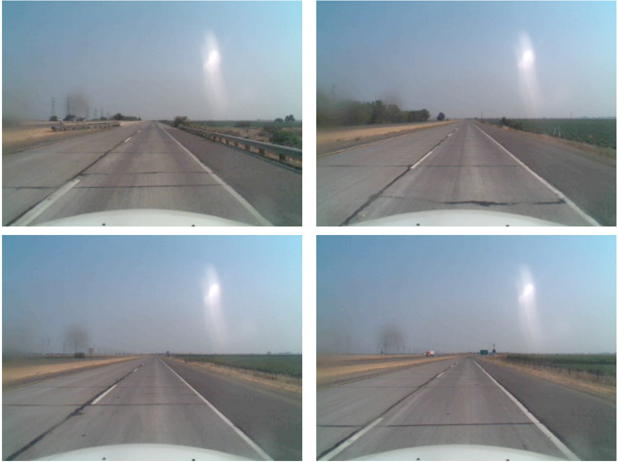
Figure B.1. View of segments A, B, C, and D on BD pavement.
