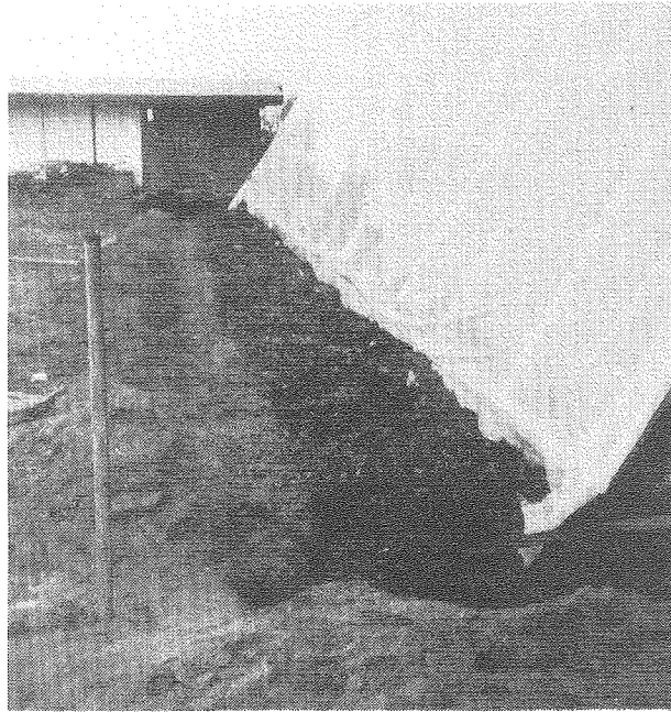
Compost pit insulation.
