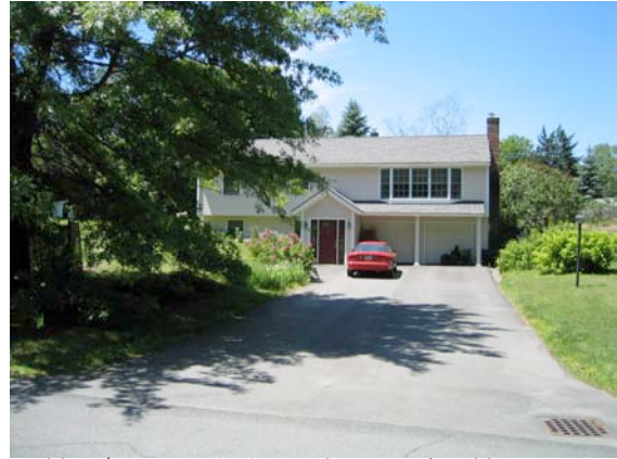
Building/Lot View A: Street Elevation of Building (#3538)
