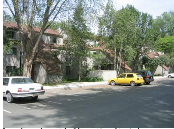
Large lot twelve-unit building with parking in front (#4303)
