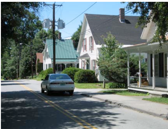
Row of small multi-unit buildings in N5 Maple (#5167)
