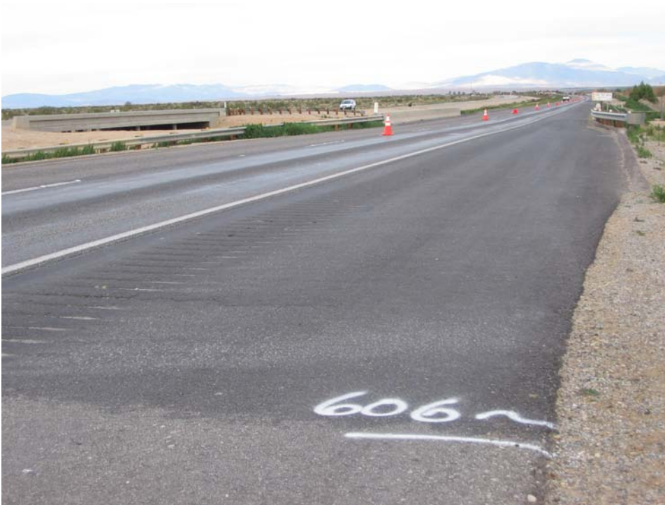
Figure 5. Station 606, facing north – RAC chip-sealed section starts here.
