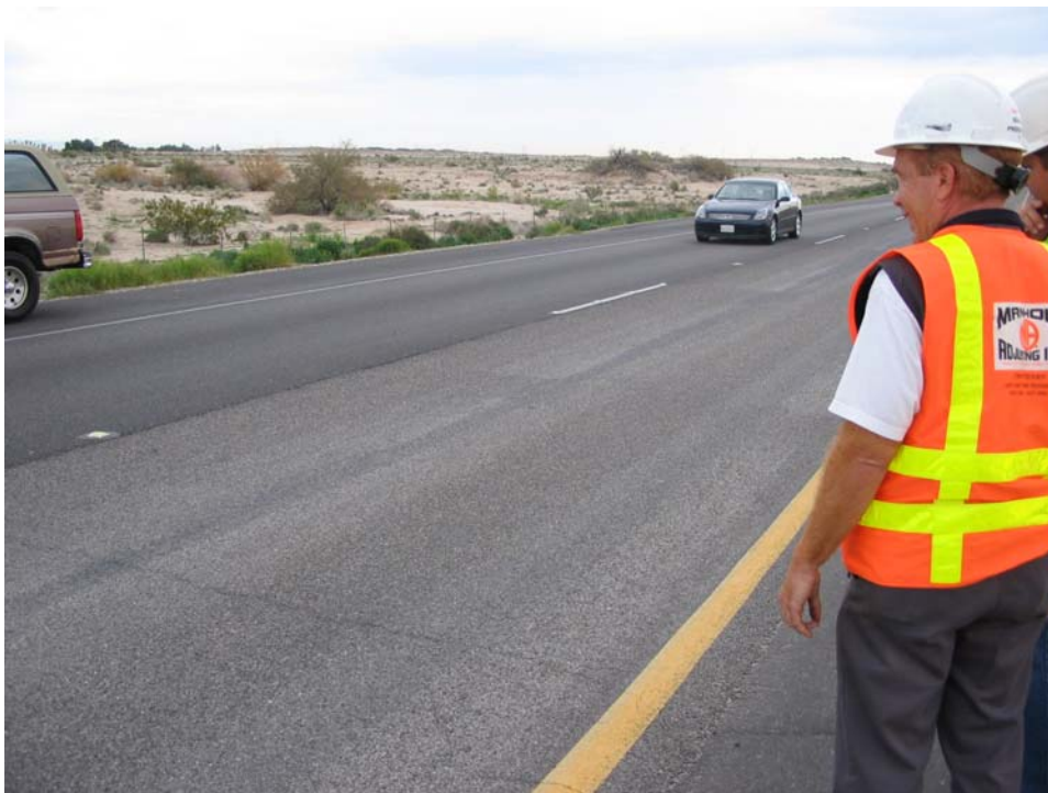
Figure 13. Station 688, facing south—OGAC + RAC chip sealed #2 lane without evidence of distress.
