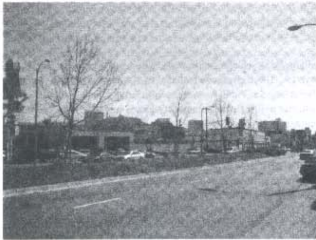
FIGURE 2 Median separation of right-of-way at San Pablo Avenue at Sycamore in Oakland; landscaped medians can be found along San Pablo in Oakland and Berkeley.
