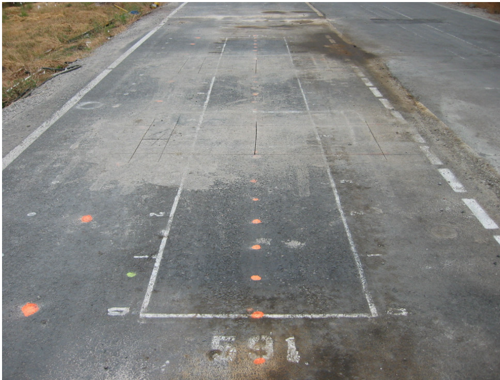
Figure 3.36: Section surface viewed from Station 0.
