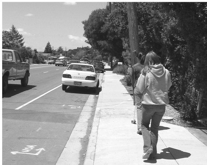
Figure 1. Example of a SR2S traffic improvement project. San Pablo Dam Road near Sheldon Elementary School before (above) and after (below) the SR2S-funded project to install new sidewalks.
