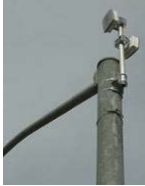
Figure 4-13: Typical WLAN Bridge/AP Equipment Installation
