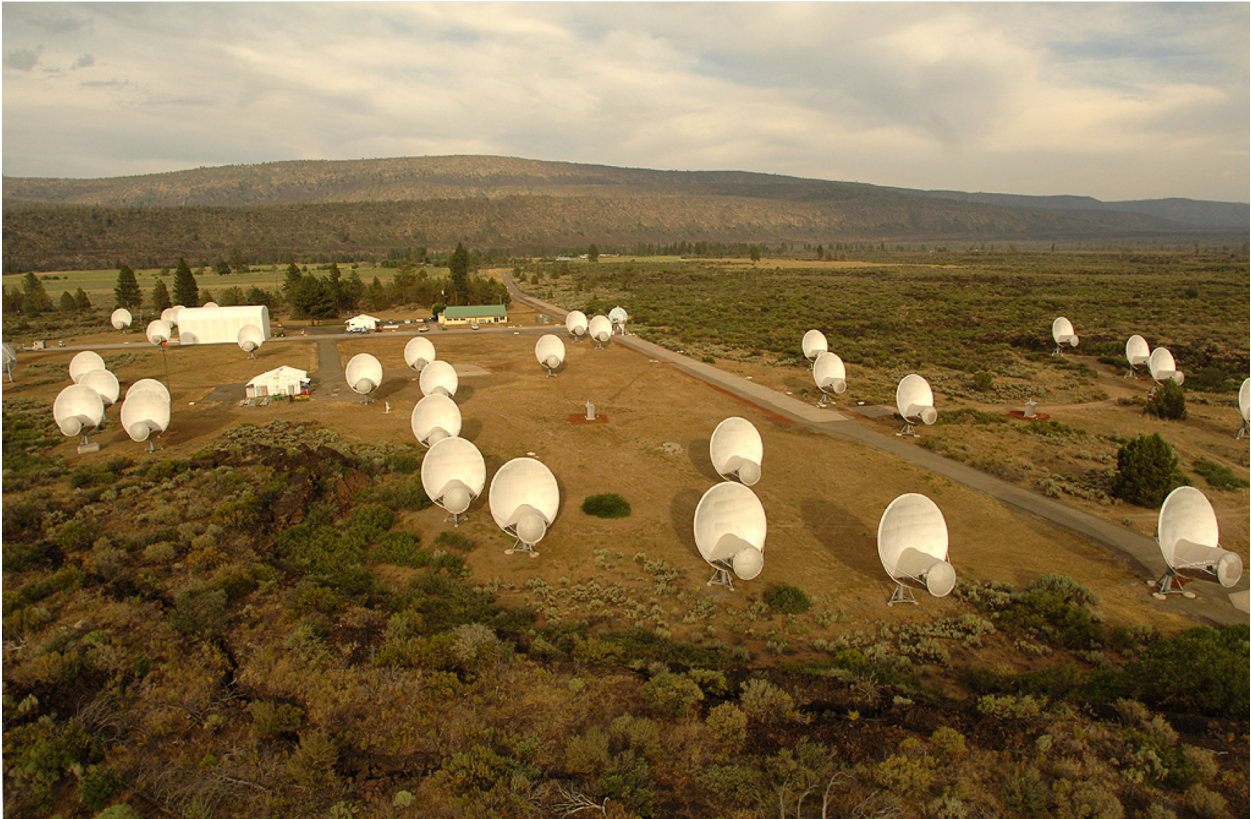
Figure 1.2: Elevated view of a portion of the Allen Telescope Array, looking approximately east. The large white structure is a tent for antenna construction, and the smaller yellow structure is the control building, housing the signal processing room and observer facilities.
