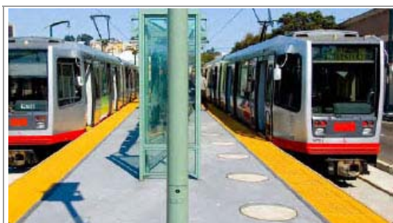
Figure 11 - Typical Muni at-grade station Source: Muni 2007b
