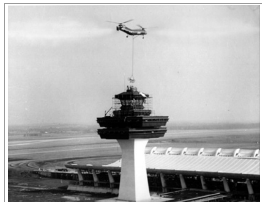
Figure 24 – Dulles construction, circa 1961 Source: http://www.faa.gov/
