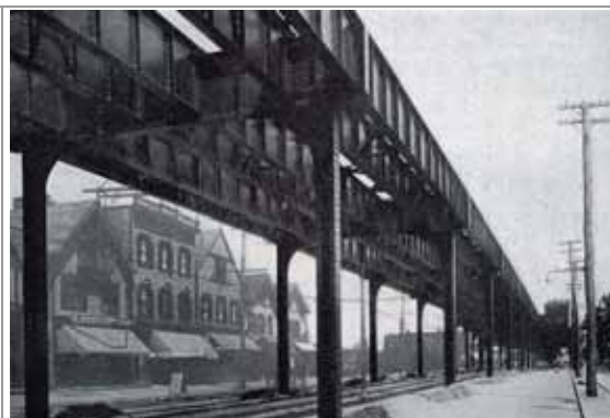
Figure 15 – New York City aerial support similar to Green Line Source: Griest 1915
