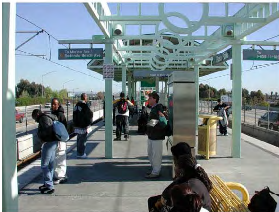
Green Line Platform in I-105 Median
