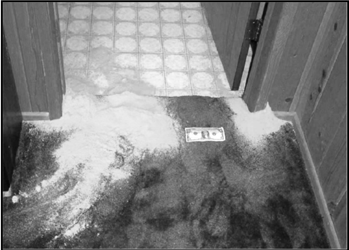
Figure 1: Insulation removed by L. luctuosum in a mountain home in the San Bernardino Mountains, CA.
