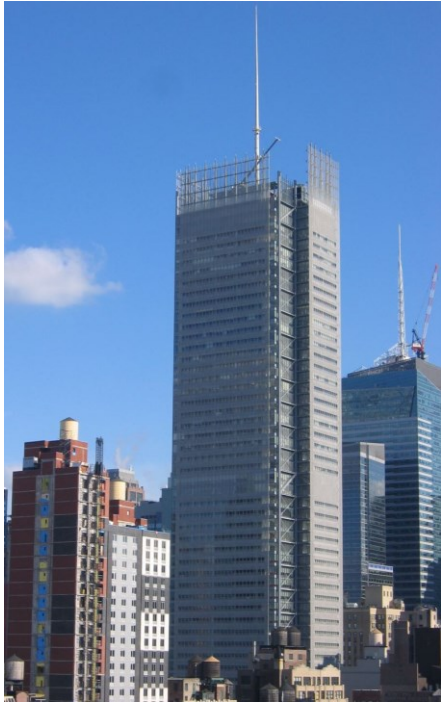
Figure 3.2.1-9: The New York Times Building
