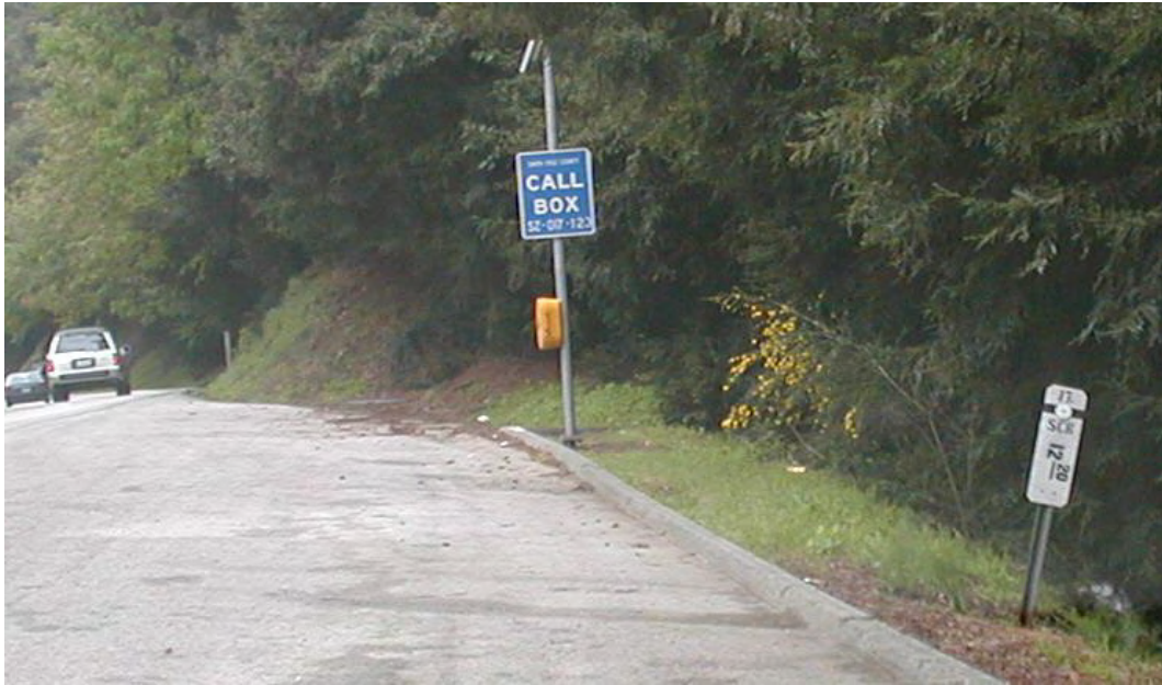
FIGURE 15. Pullout with motorist call box and post mile marker.
