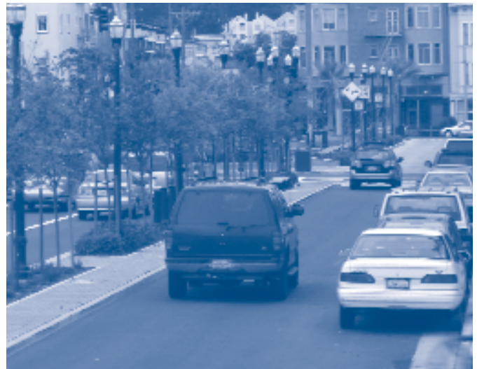
Too-wide side access roadways
