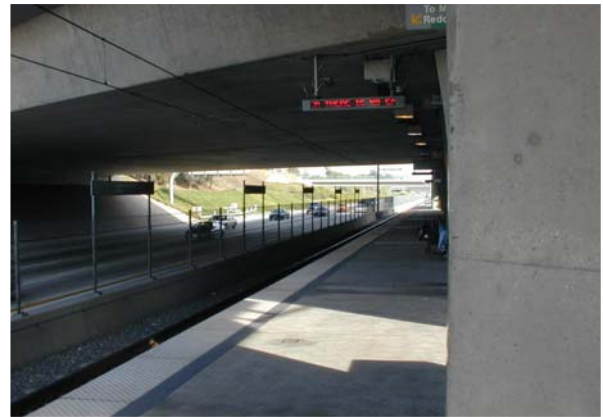
Figure 5: Underpass Platform at Lakewood Station
