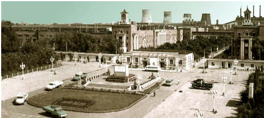
Fig 5-3 the bird view of the main gate of the FAW in 1957
