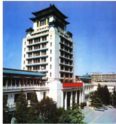
Fig 5-5 National Cultural Palace in Beijing, designed by Zhang Bo in 1958
