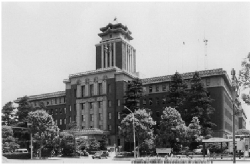
Fig 2-1 the Kanagawa Prefectural Office Source: Jonathan Reynolds, p.91
