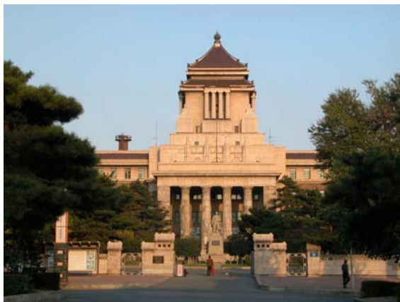
Fig 3-7 the building of colonial State Department, built in 1933
