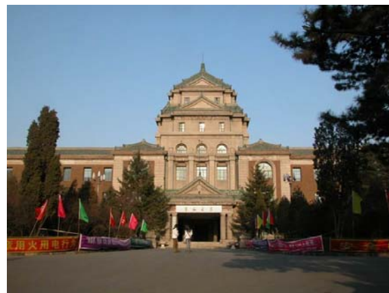
Fig 3-8 the building of colonial Ministry of Justice, built in 1934
