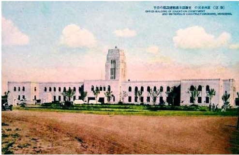
Fig 2-5 the CCB building at Datong Plaza Source: Li Zhong, p.144
