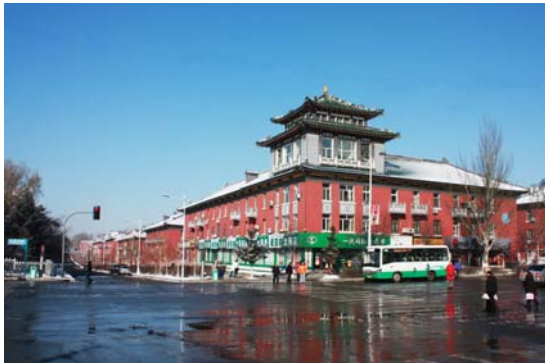
Fig 5-15 view of the towered residences. Its ground floor is still used for shop.
