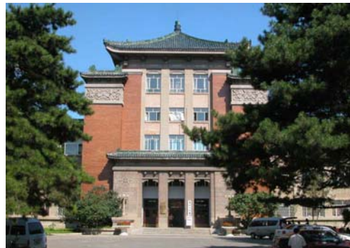
Fig 4-17 The Provincial Library built in 1957, four blocks from the Palace of Geology
