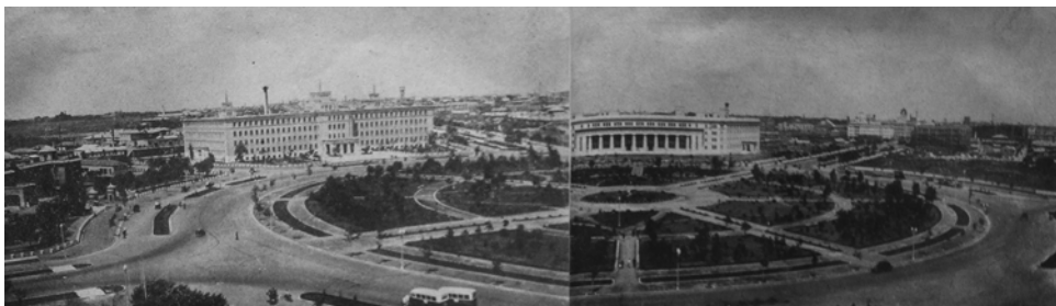
Fig 1-6 Datong Plaza under construction, 1933
