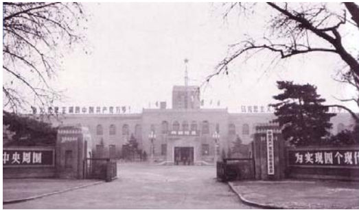
Fig 4-7 The former CCB building was reused for people's Municipal Government of Changchun
