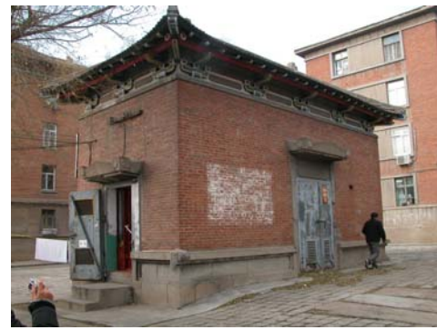
Fig 5-16 an electric distribution station within a Chinese-style housing block
