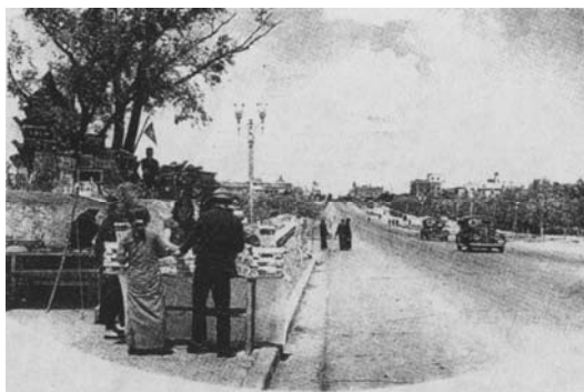
Fig 1 Xiaoqifeng at Datong Street with the railway station in the far background. Note the intrusion of the temple into the street.
