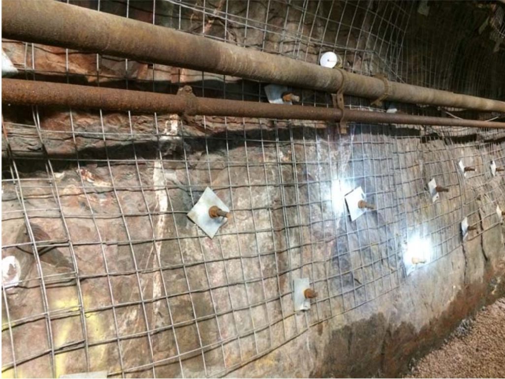
Figure 2.4. Veined and sheared amphibolite that corresponds to a zone of decreased seismic velocity between the East and West Access Drifts near Drill Stations 1 & 2.
