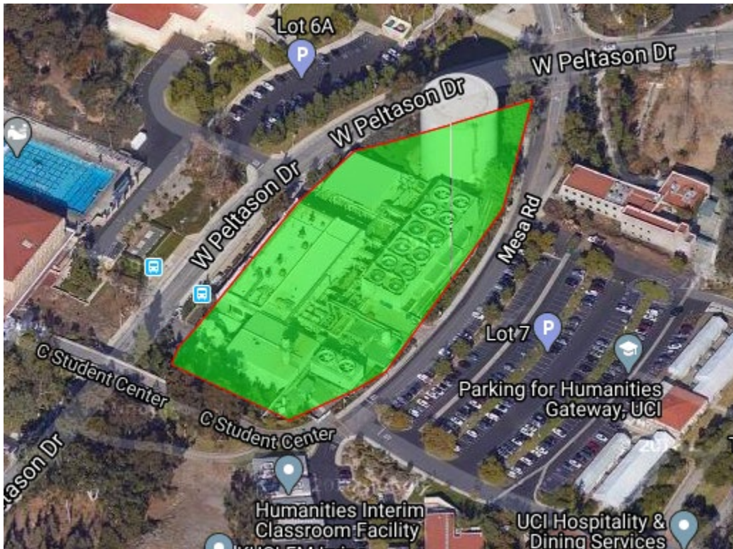
Figure 32 – Overhead view of UCI’s central plant area, the highlighted area being roughly 9500 square meters.
