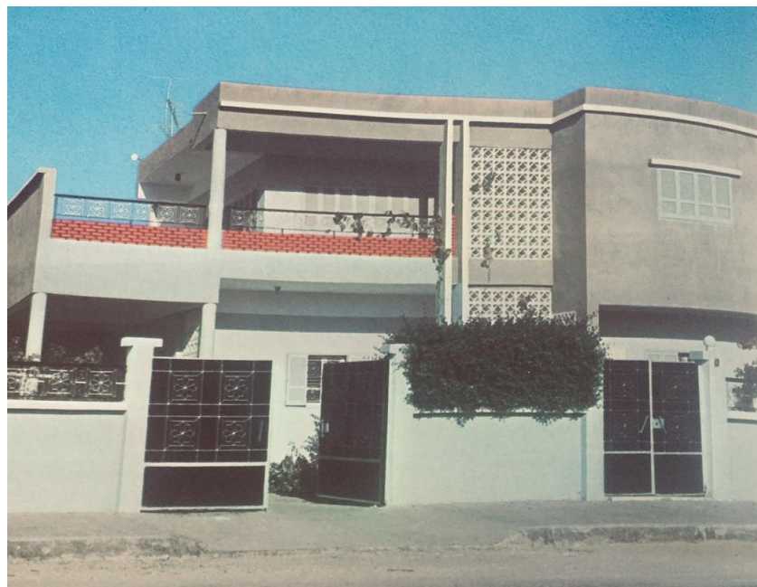
Fig. 2-12: A villa built using the Aramco homeownership program. Source: Twitter.
