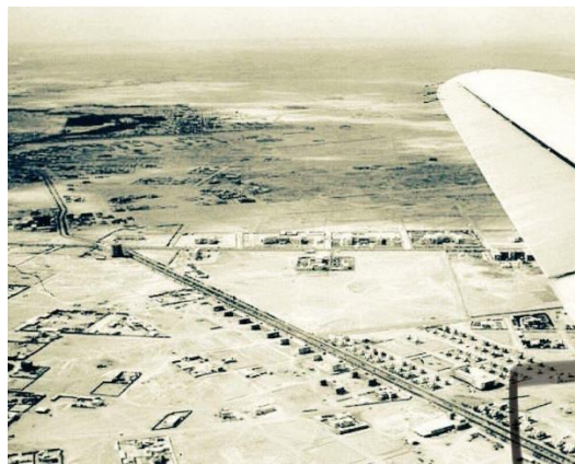
Fig. 2-14: An aerial image of Al Malaz during its early construction. Source: Al Assaf twitter (@Mansoralassaf).
