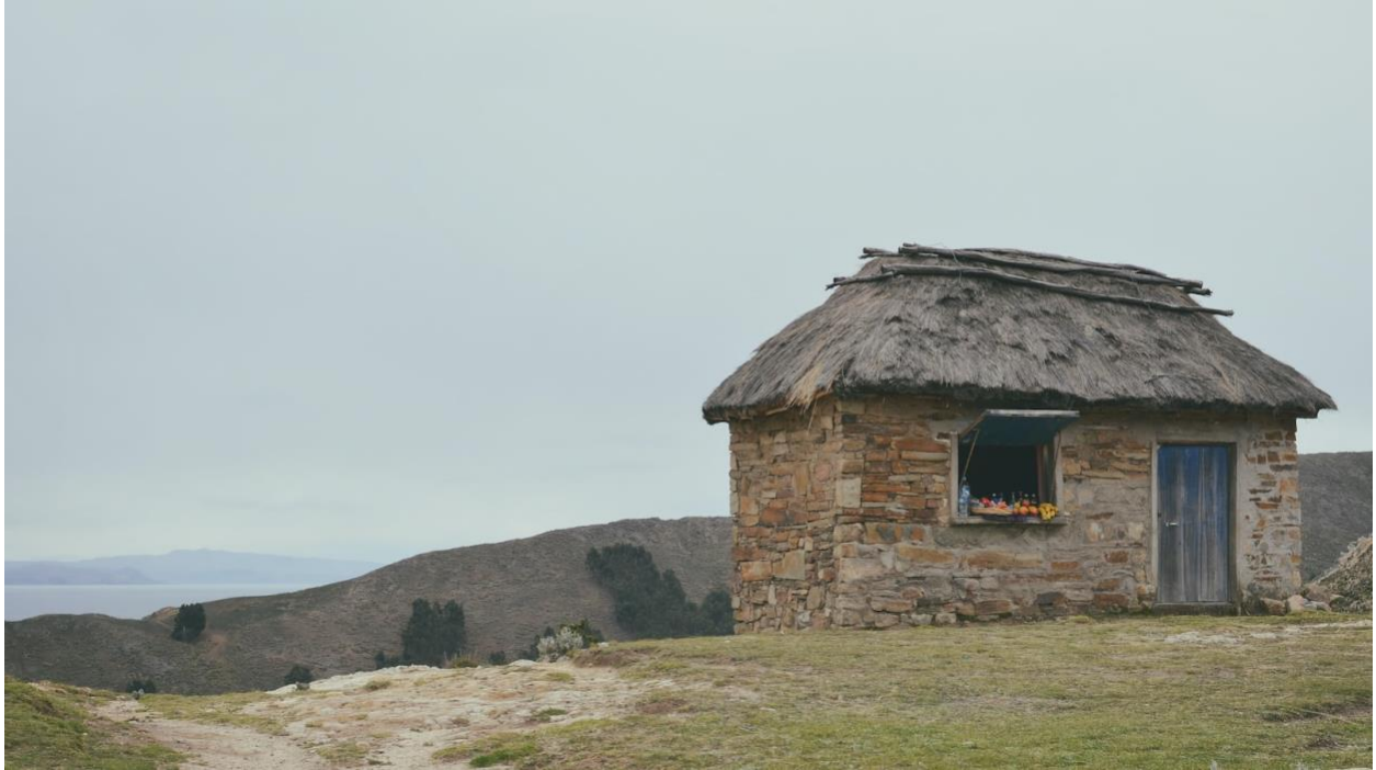
Figure 19. Example of a thatched roof on present-day Aymara architecture, Bolivia-Peru border. Photograph by Paz Arando, 2016, brown brick house , Unsplash, accessed June 11, 2023, https://unsplash.com/photos/fpw2EF6W_NY .
