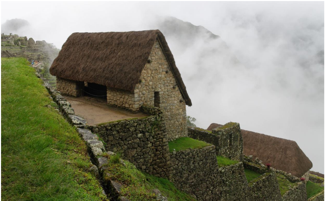
Figure 20. Photograph of an Inca thatched roof reconstruction in Machu Picchu, Peru. Photograph by Emmanuel Dyan, 2010, Machu Picchu, Inca Trail (Fourth Day), Peru , Flickr, accessed June 13, 2023, https://www.flickr.com/photos/emmanueldyan/4289678266 .
