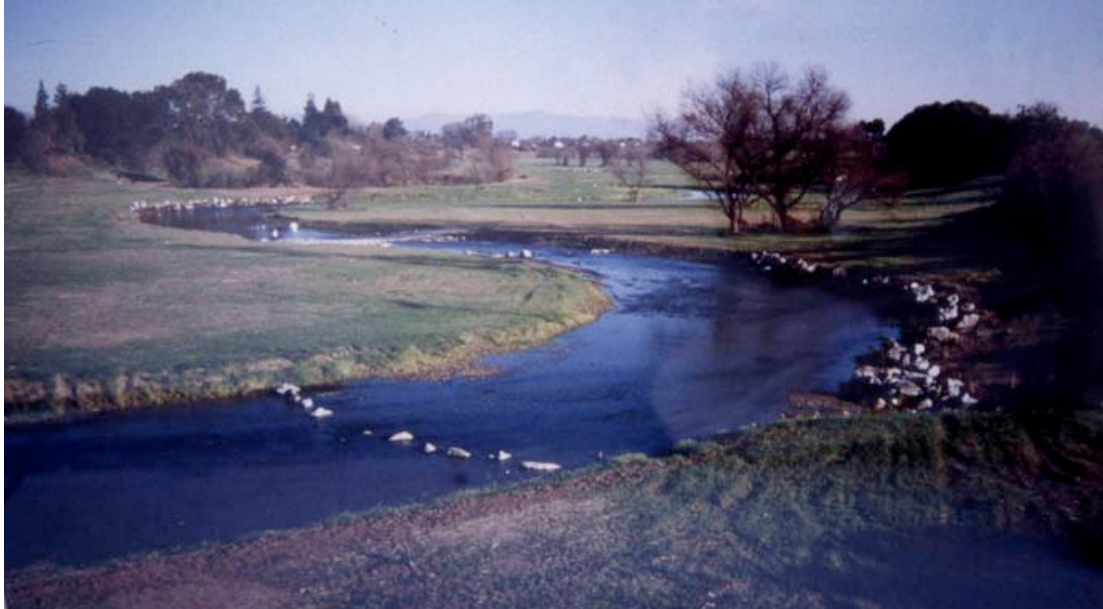
Figure 13. Uvas Creek restoration with armoring on the outside of the bends and rock weirs spanning the channel in January 1996, two months after construction (City of Gilroy, from Kondolf 2006).
