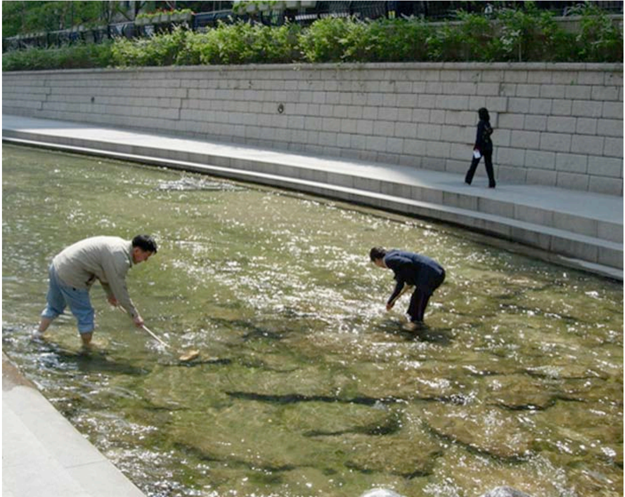
Figure 27. Workers scrub the algae off the rocks and bottom of the Cheonggyecheon (François Rejeté).
