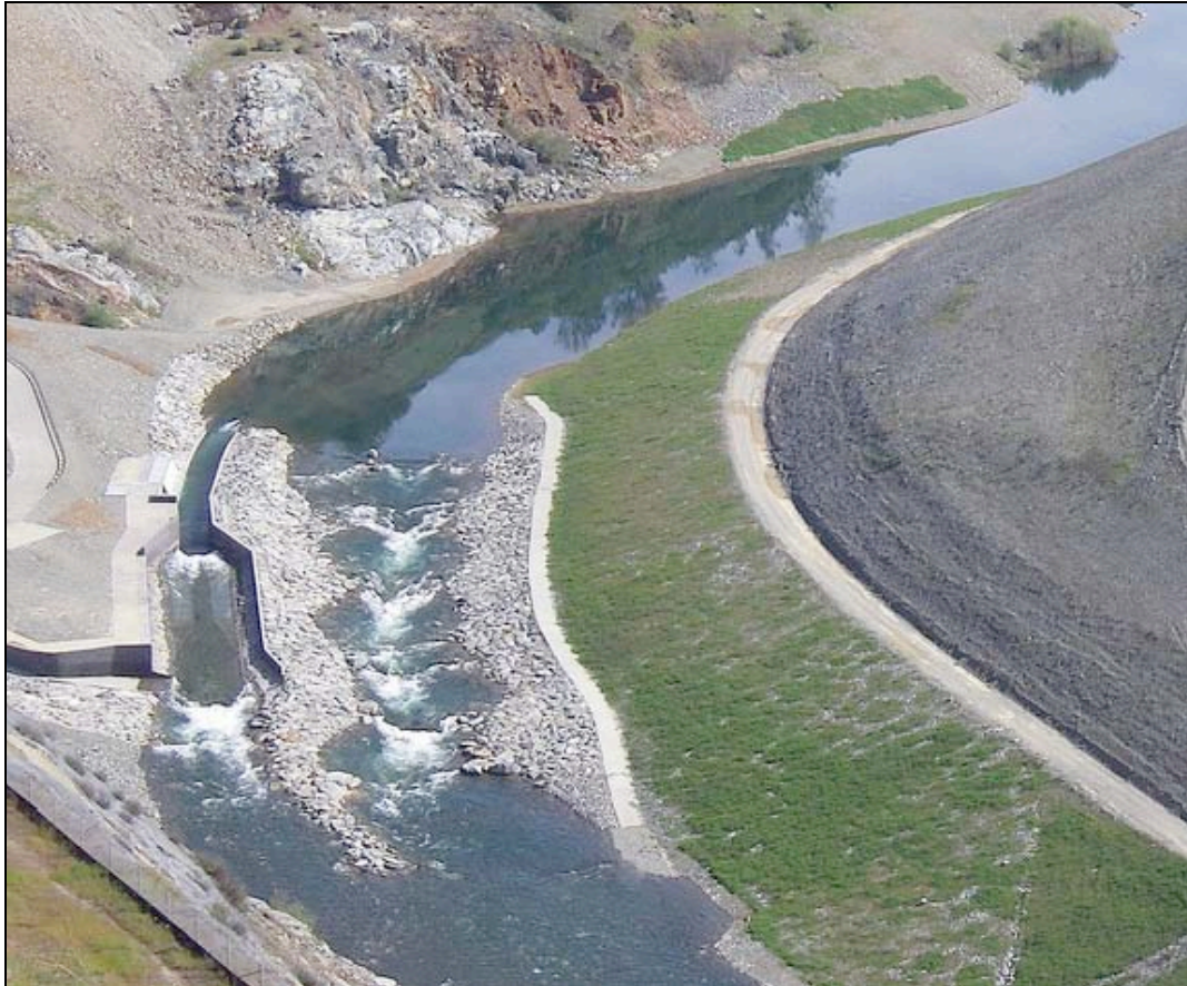
Figure 39. A multifunctional fish passage, water diversion, and whitewater design on the American River in Auburn, California. The whitewater channel or hydraulic chute channel is to the right in the image. Photo compliments of McLaughlin Water Engineers.
