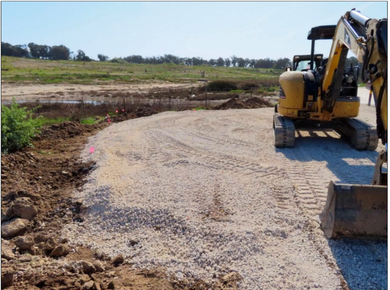
Overlook under construction on the Marsh Trail.
