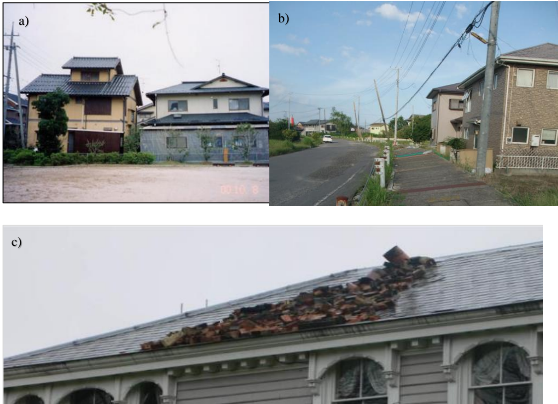
Figure 4: Structural damage due to liquefaction: (a) Tilting of a house, (b) Tilting of a house in Hinode, Japan, (c) fallen chimney bricks, (Ishihara 2011, Buchanan et al. 2011)
