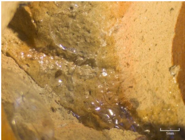
Figure 9: The adhesive has become brittle and joints are failing.
