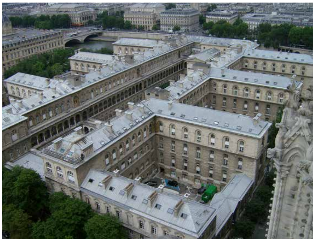
Fig. 34. Hôtel-Dieu, Paris, the oldest existing hospital in the world. It was largely rebuilt after a fire in 1772. As part of a hospital reform movement, its winged wards were designed to increase air flow, providing better conditions for the large volume of patients in the teaching hospital
