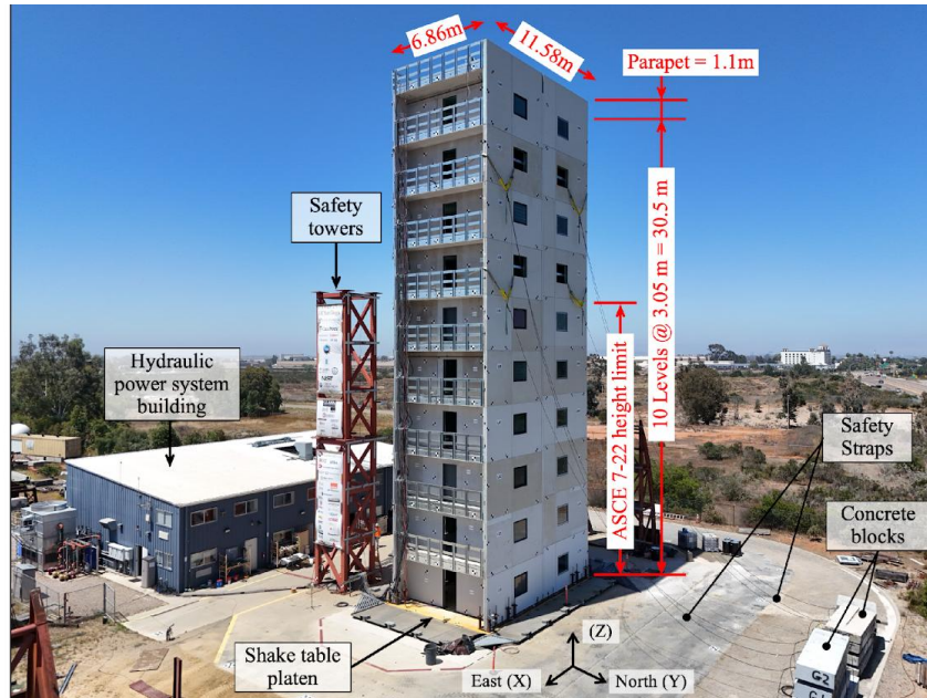
Figure 4. Northeast view of the CFS10 specimen with annotations (Hutchinson et al. 2026).
