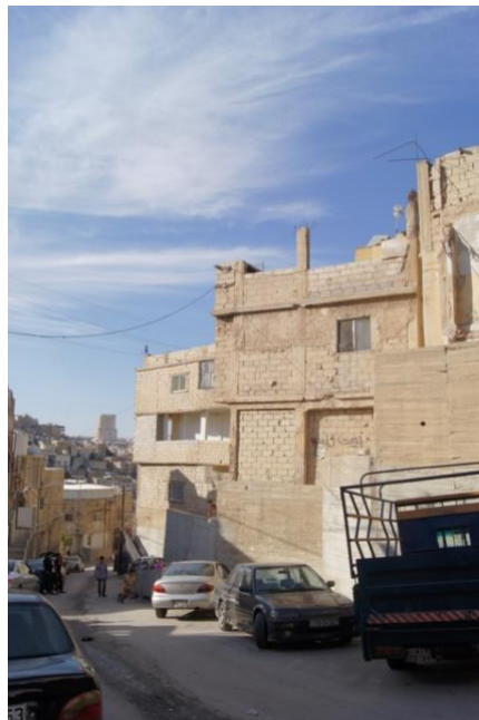
Figure 3-8. The Visual Remains of Demolition – Outlines of Room Cut in Half, Broken walls, and Hanging Ceramic Tiles. Photos by author.
