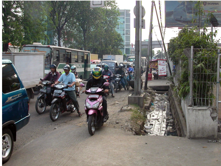
Figure 11: A cart-pusher meanders between poles and competes with motorbikes and trucks using the unpaved shoulder of Jalan Daan Mogok, West Jakarta
