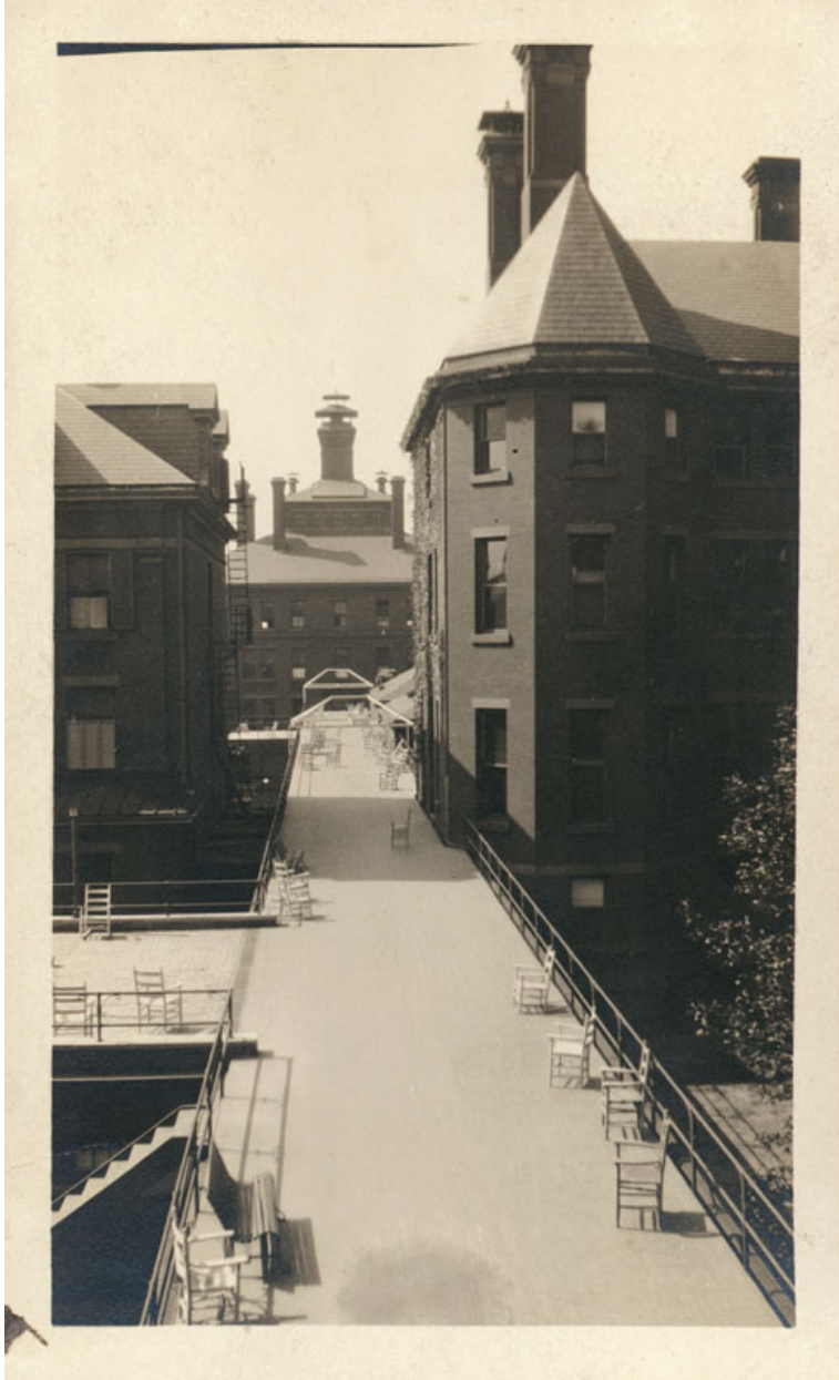
Figure 1.16: View of Open Terrace Walk between the Administration Building and the Annex, Johns Hopkins Hospital, circa. 1900, Alan Mason Chesney Medical Archive, Johns Hopkins Medical Institutions, item 148166.
