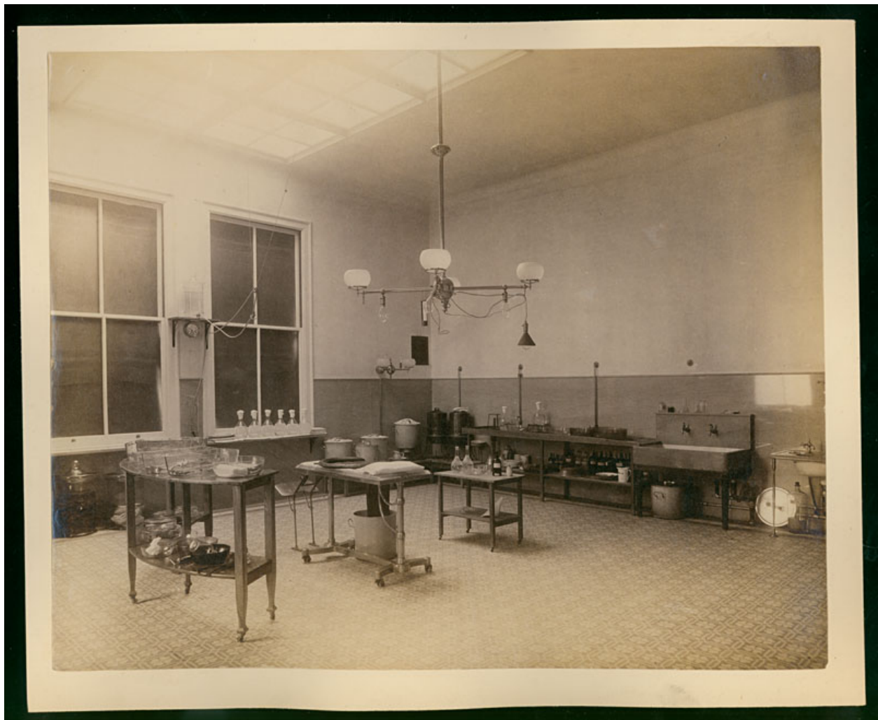
Figure 3.35: Gynecological Building operating room (1892), Buildings Photograph Collection, Alan Mason Chesney Medical Archive, Johns Hopkins Medical Institutions
