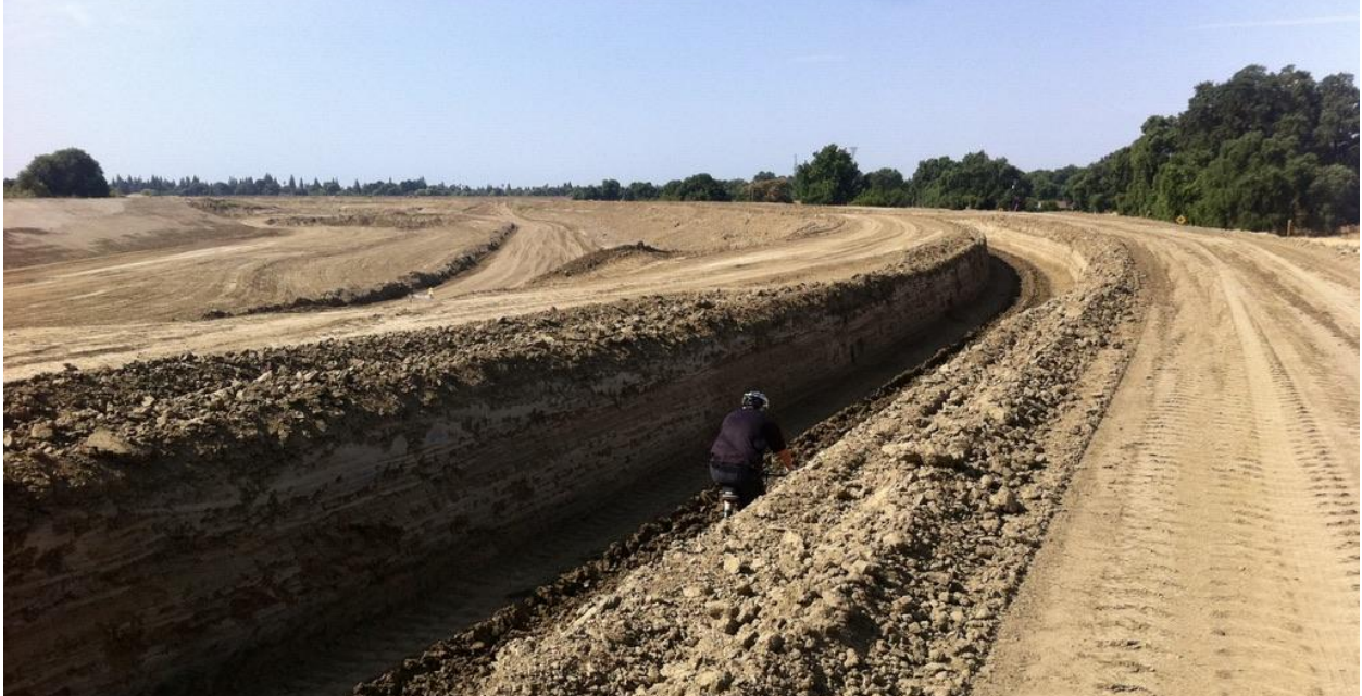
Biking in the levee. Near northern breach site. July 22, 2018
