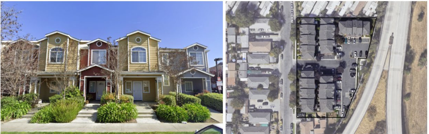
Figure A7.10: Townhouses can be connected in linear fashion, but designed to express the individual units; 745 Bonita Place. San Jose, CA.
