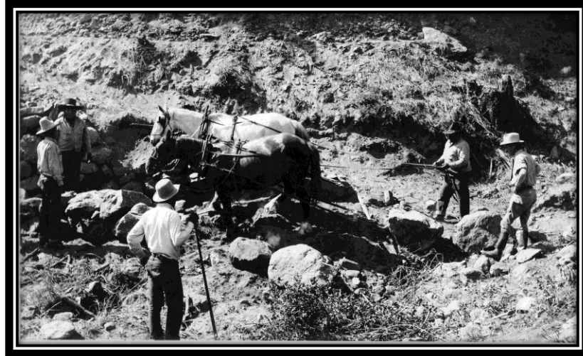
Photograph 1. Cutting the road on the Santa Ysabel Indian Reservation with horses and plow (c. 1937). From the Records of the Bureau of Indian Affairs, Record Group 75, National Archives Pacific Region (Laguna Niguel).
