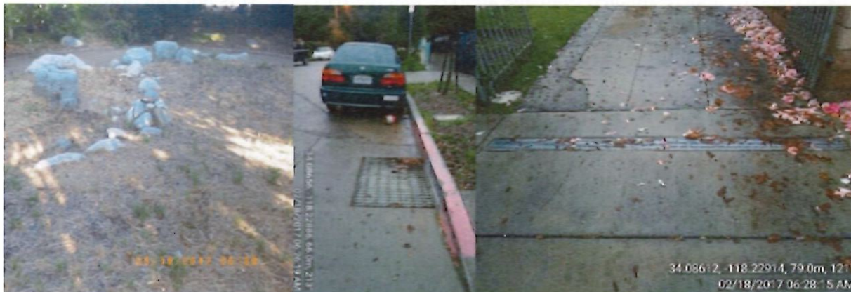
Figure 12. Oros Green Street Vegetation/Infiltration Trench Drain Inlet/Driveway Trench Drains.
