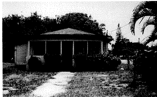
Typical shotgun and "cracker" houses in the Mount Olive neighborhood, Delray Beach, FL.
