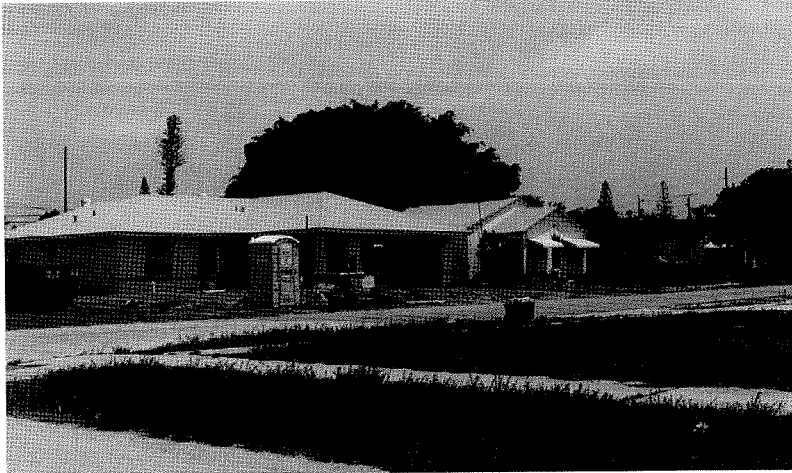
Above and opposite page: Typical new construction in Mount Olive.
