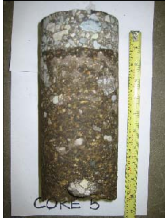
(b) Core 5 taken from the southbound lane
