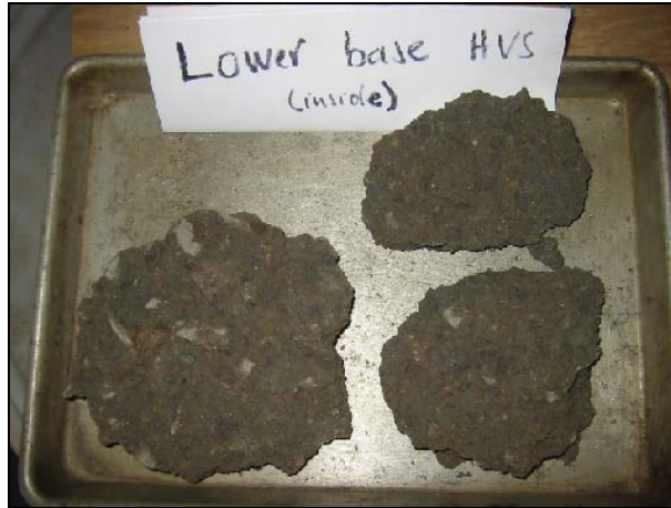
Figure 4.24: Flaky, clay like material from below the base layer on Section 593FD.
