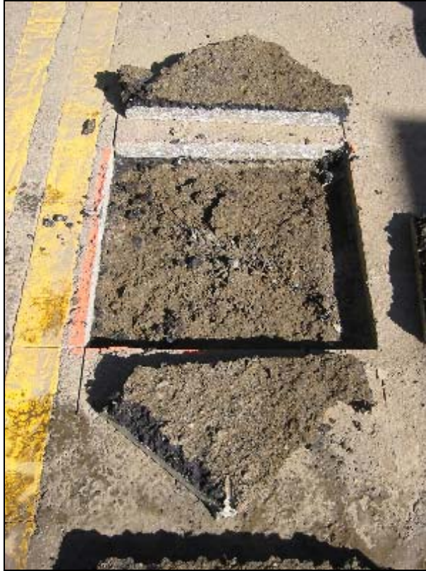
Figure 4.19: Asphalt concrete surfacing removed from the test pit on the mainline.
