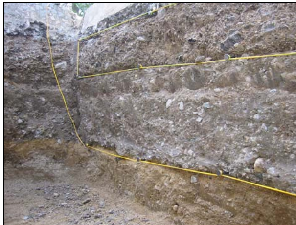
Figure 4.25: Test pit Section 593FD after HVS trafficking.
