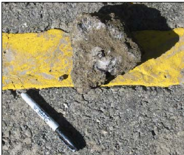
Figure 4.20: Intact piece of reclaimed asphalt concrete found in the mainline test pit.
