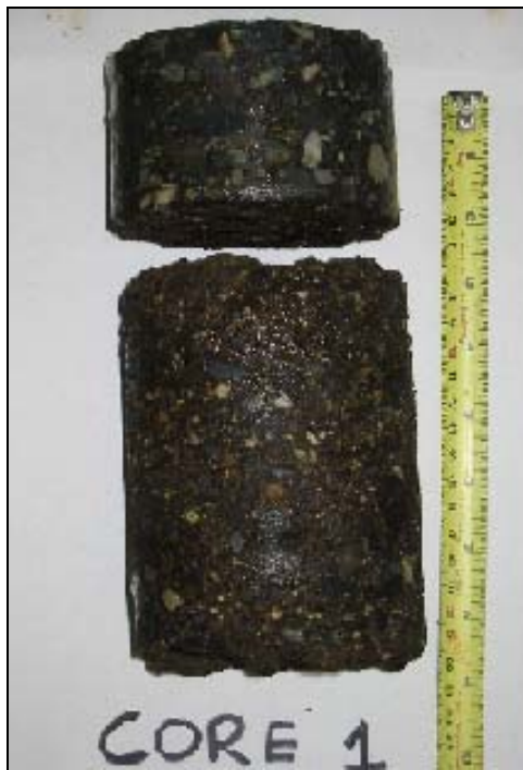
(a) Core 1 taken from the northbound lane
