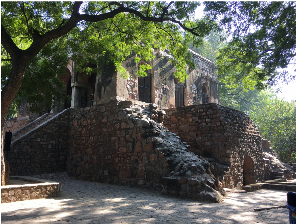
Figures 2.20, 2.21 above: Nehru Planetarium designed by MM Rana, New Delhi below: Adjacent ruins of a 14th century hunting lodge
