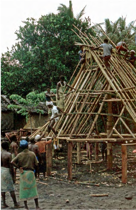
Fig. 24. Construction of the naulum roof. Potne village, Kilenge, West New Britain, Papua New Guinea, c. 1977. Photograph courtesy of the author
