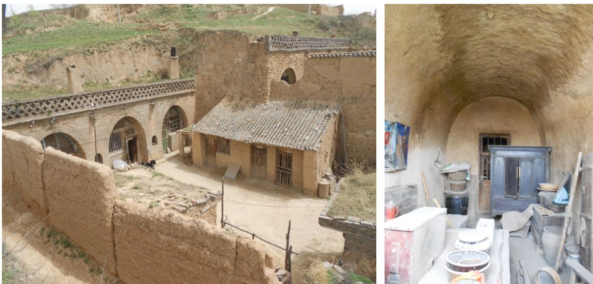
Figure 68. Left, typical Shanxi residence with arcuated rooms, known as yaodong , cut 5-8m into the loess soil; right, interior of one yaodong in the countryside around Pingyao.
