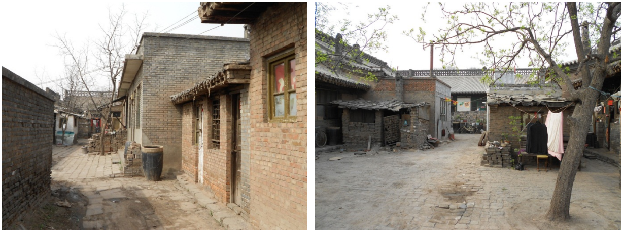
Figure 71. Left, multiple new structures within Fanjia Jie courtyard house; right, compound with multiple additions (note integration of older grey brick with newer red brick)
