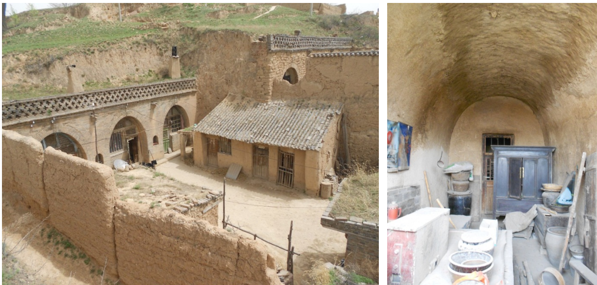
Figure 68. Left, typical Shanxi residence with arcuated rooms, known as yaodong , cut 5-8m into the loess soil; right, interior of one yaodong in the countryside around Pingyao.
