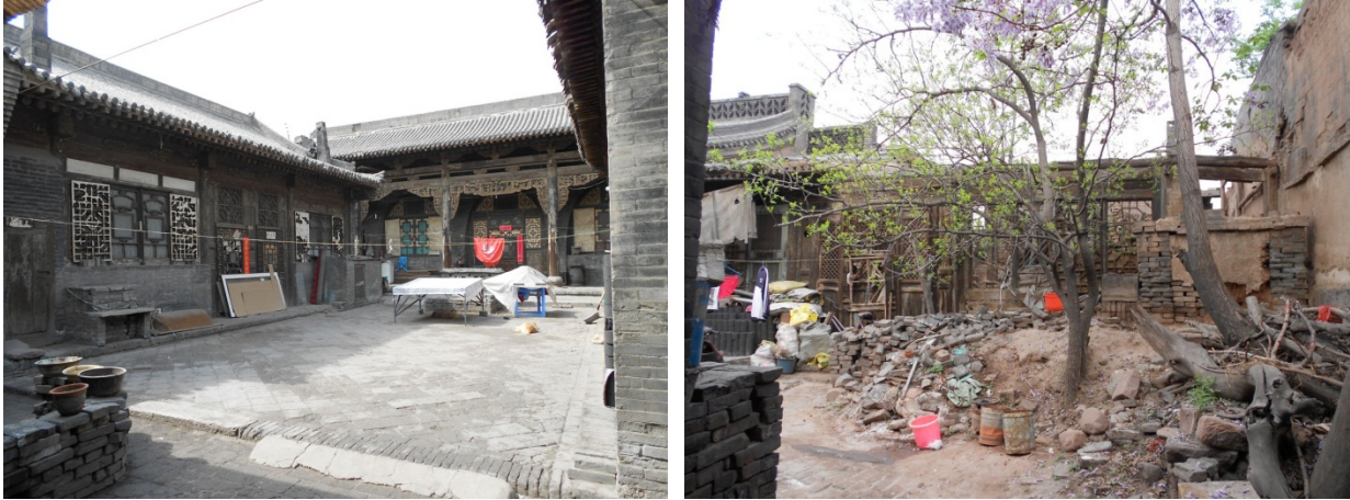
Figure 70. Left, Fanjia Jie courtyard house in good state of preservation, with intact decorative woodwork; right, Shaxiang Jie courtyard house structure with only wooden façade of extant (behind tree)
