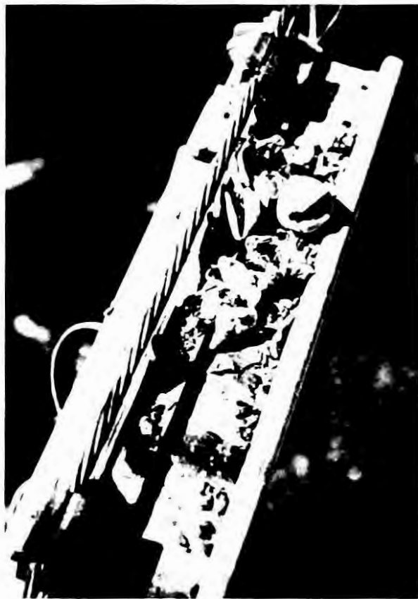
Figure 4. Gnawed almond shells and rat droppings on top of the terminal shown in Figure 2.
