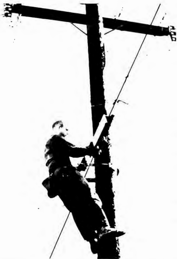
Figure 2. Diphacin bait blocks being attached to a utility pole above the telephone cable. The terminal is adjacent to the workers right arm.
