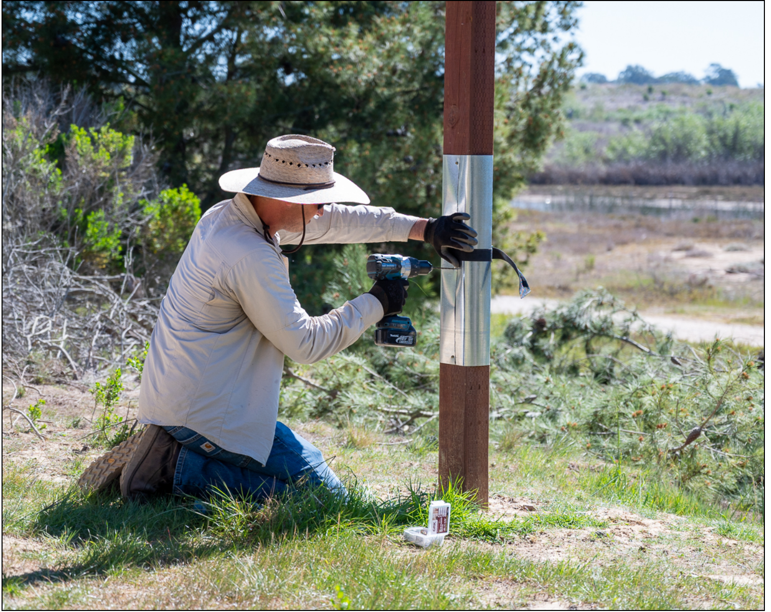
NCOS Manager Darwin Richardson installing the metal wrap.
